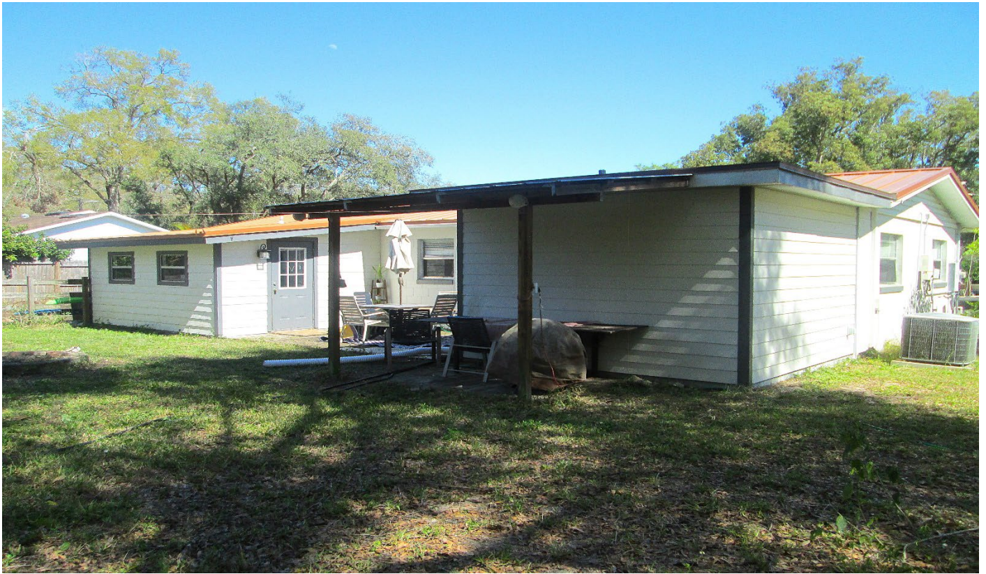
Rear yard, facing northeast towards existing rear of residence
