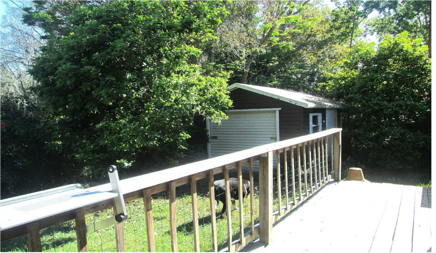
Side yard, facing southeast towards existing accessory structure
