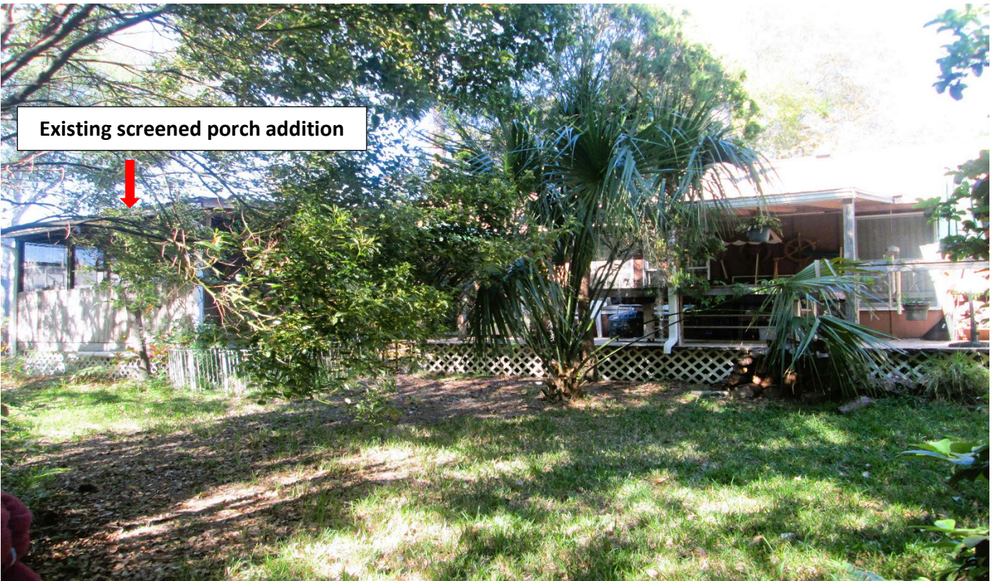
Rear yard, facing northwest towards existing rear of residence
